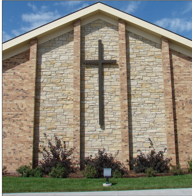
The soaring brick and stone with a simple cross provides a solid, yet dramatic look to the new addition.
